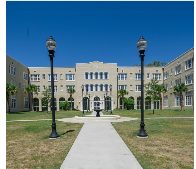
Hardy Hall Courtyard
