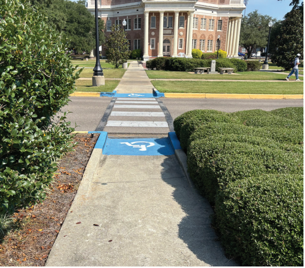
Enhanced pedestrian crossing on Southern Miss Drive
