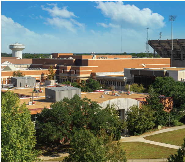
Walker Science Hall (renovation proposed)
