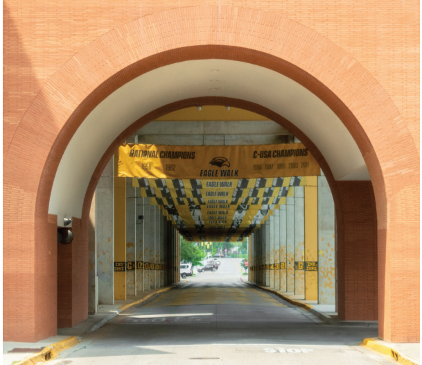
Eagle Walk Tunnel
